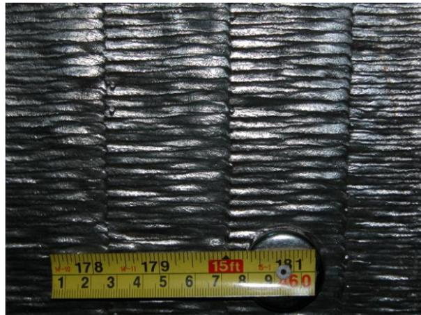
Figura 3.25: *weld overlay* vertical acabado (Wensley, 2004).
